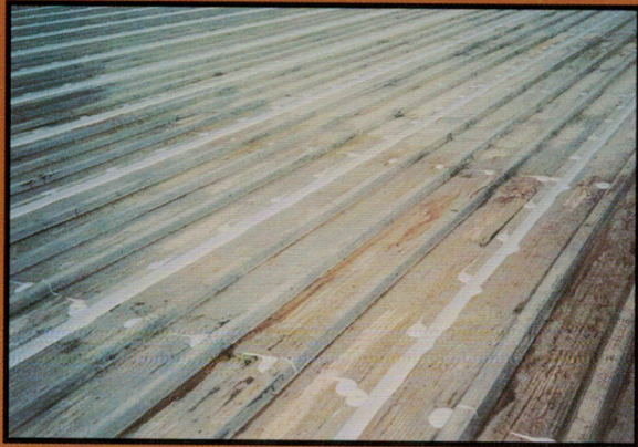
Truco's Eterna-Seal® Super seam sealer is applied to all seams and fasteners.
