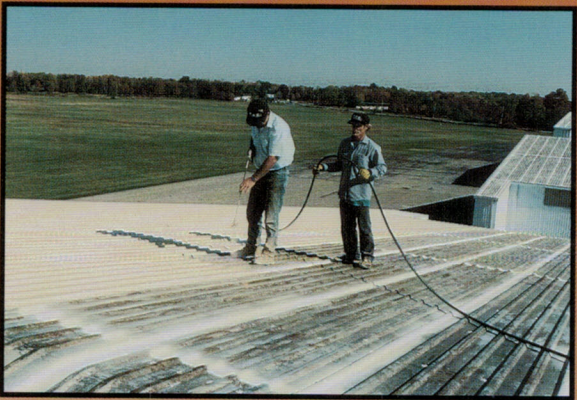
First coat of Truco's Eterna-Seal® rubber coating being applied with sprayer.
